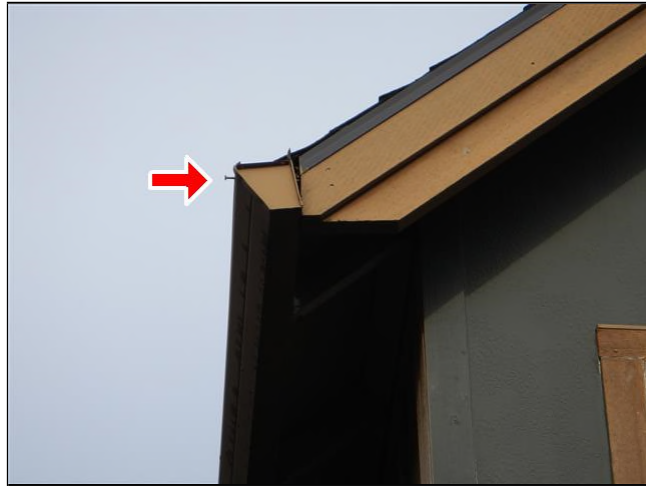
Spike protruding out needs to be tightened in order to keep gutter against fascia and water away from house.
