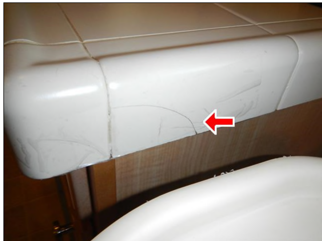
Small hairline crack in kitchen countertop.
