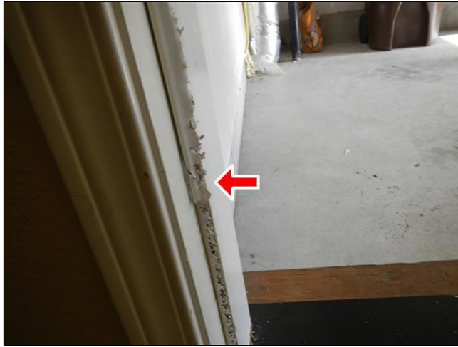
Weather strip, on garage door needs repair.
