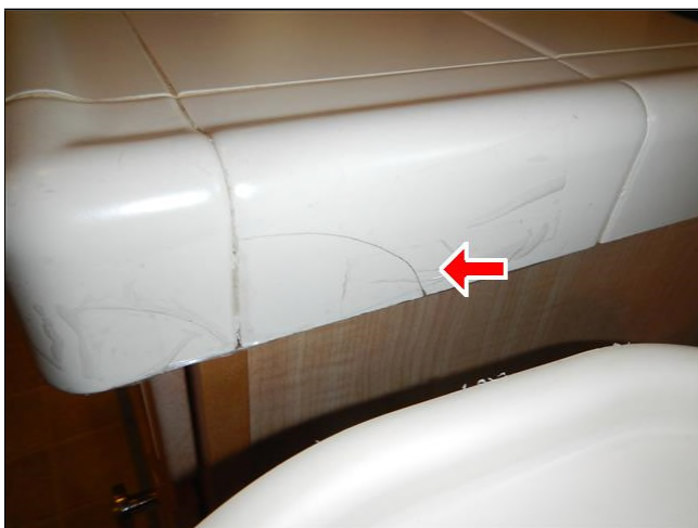
Small hairline crack in kitchen countertop.
