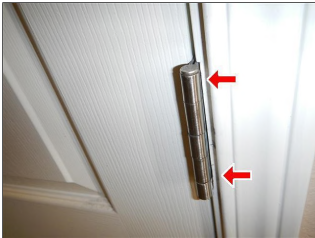
Bottom hinge needs repair. Screw is loose and needs a longer bigger screw in place.
