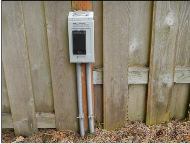
Oudoor 50 amp breaker for Hot tub.
