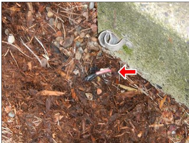
Dead wires coming out of ground in backyard for previous hot tub.
