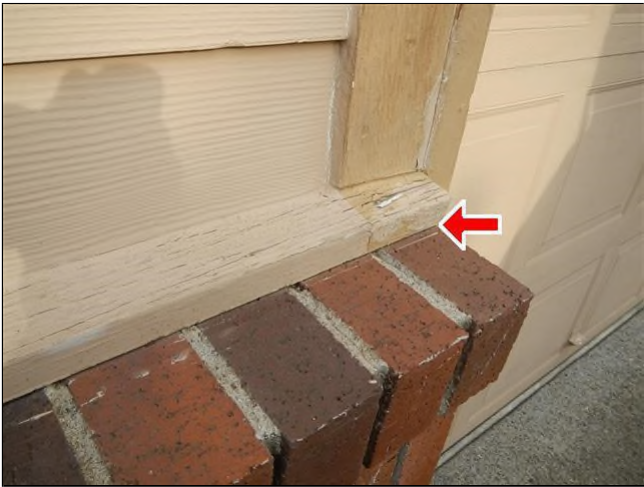
Paint needed on exterior of house to prevent water damage.
