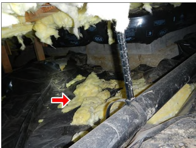
Some insulation has fallen, needs to be removed in order to prevent habitable locations for pests.
