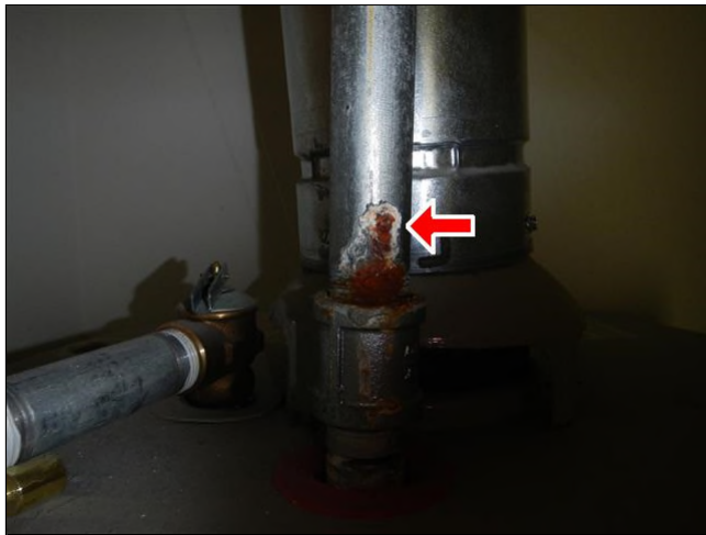
Small pin hole leak needs repair.
