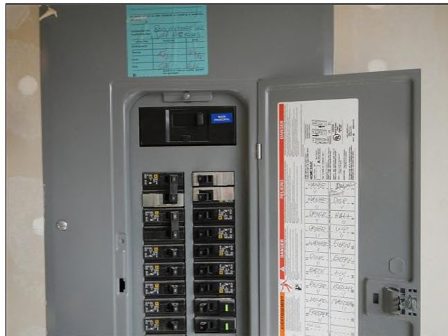
Properly labeled 200 amp Main Panel
