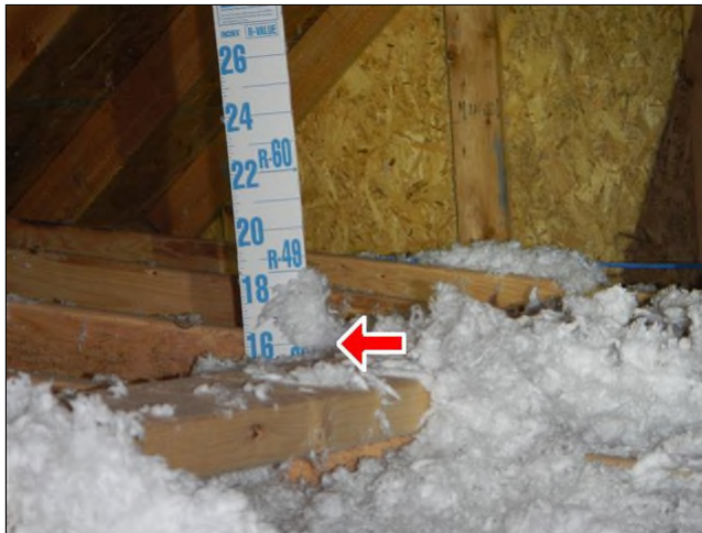
Good insulation in attic
