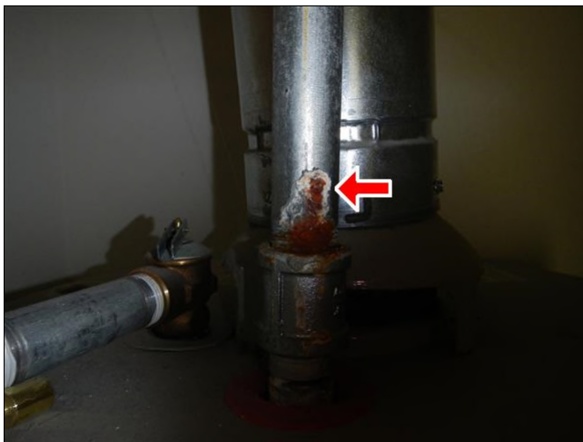
Small pin hole leak needs repair.
