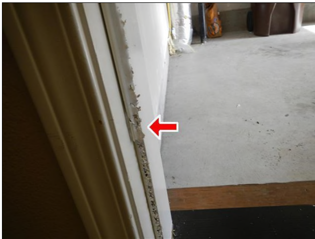
Weather strip, on garage door needs repair.
